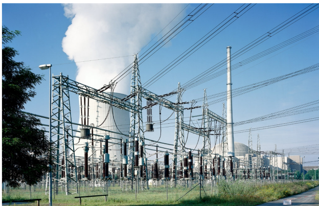
Fig. 1 The picture of a high voltage transformer substation
